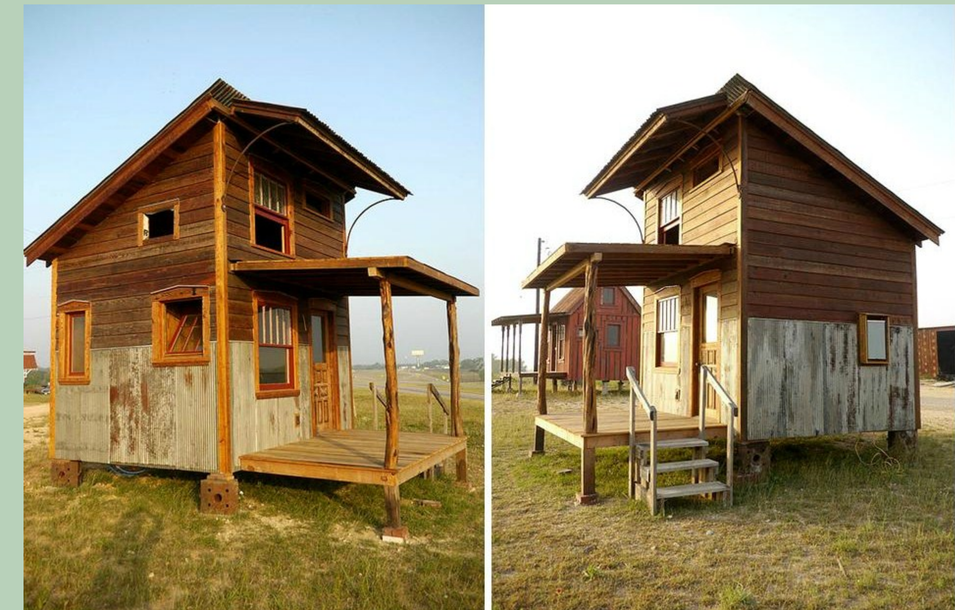
This home, built by Texas Tiny Homes, utilizes recycled construction materials salvaged from deconstructed buildings.
