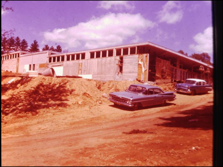
Prep School Construction- Walls Almost Done 1962 April 1962 from SJAA
