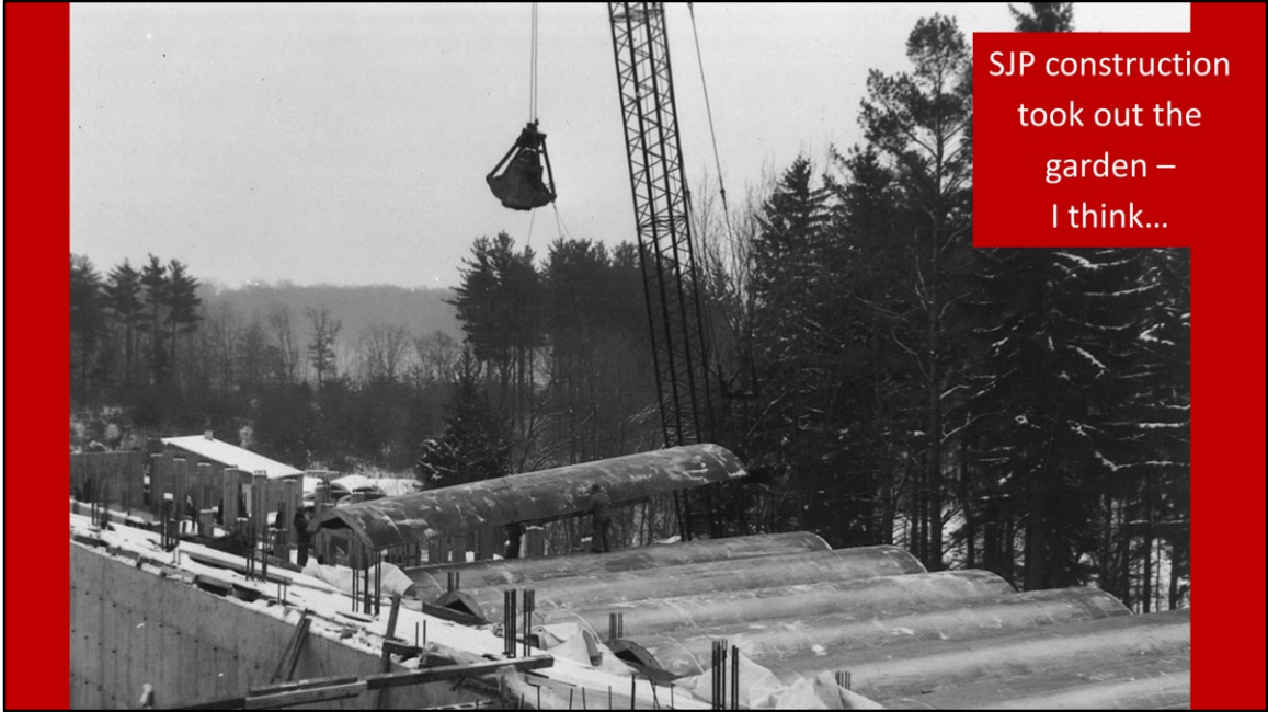
Photo of SJP construction with heavy moving equipment
