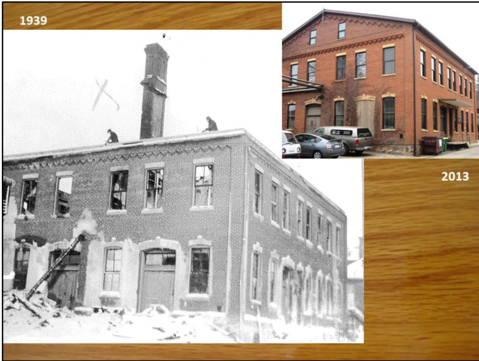
Fire damage in 1939, compared to 2013 Fire photo from Abbey Woodworking/Abbey Archives Inset photo by the archivist
