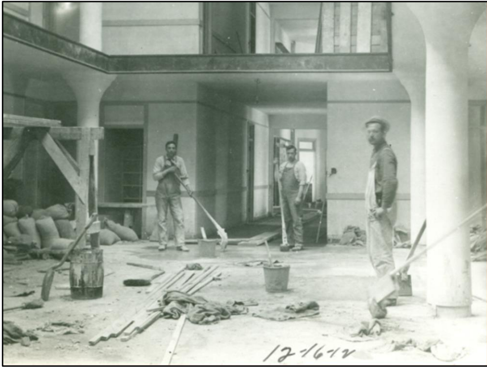
The Rotunda (Teresa Hall's 3 rd and 4 th floors) under construction
