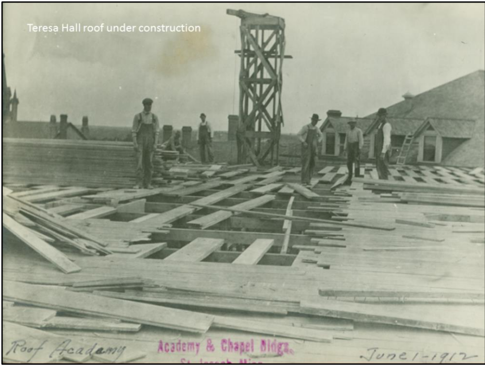
Teresa Hall roof under construction
