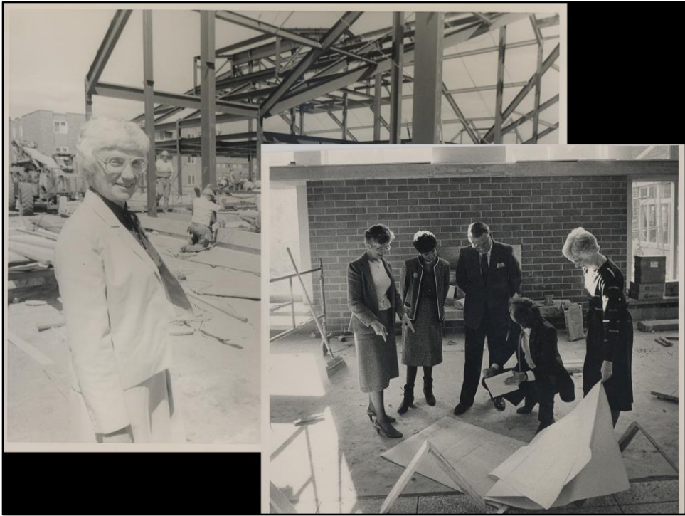
1985: Library construction is underway
