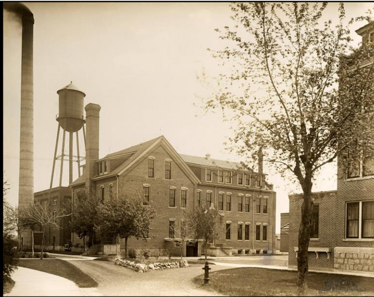
With a new power plant in place, the former power house, Loretto, was renovated and rented to the college for the Education Department and, as enrollment grew, student housing.
