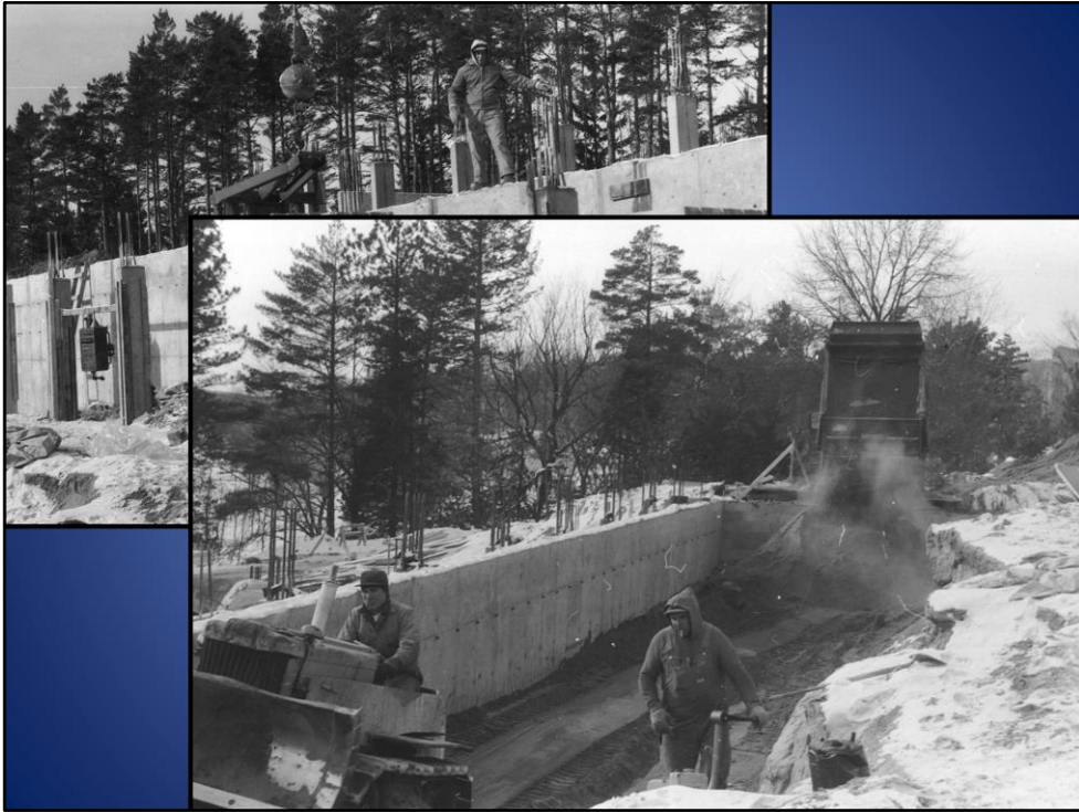
Cement work continues through the winter cold.
