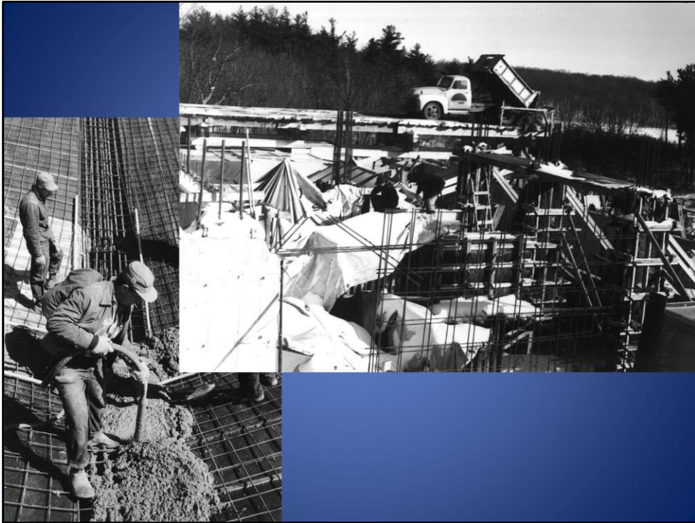
Lots of rebar, lots of cement.
