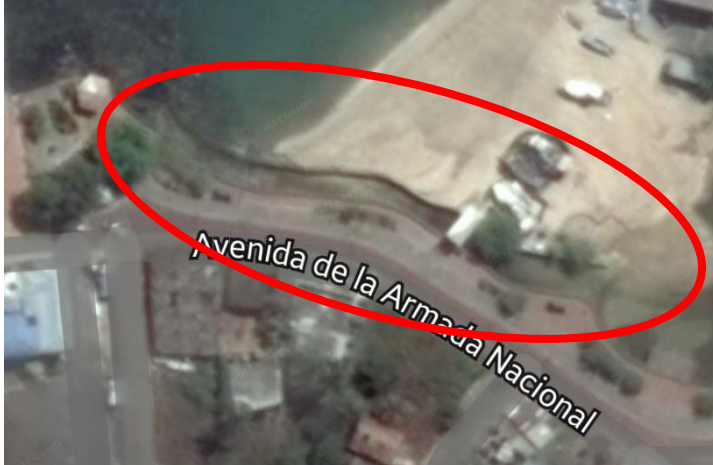
Figure 1. Ariel view of the repair beach and the tidal creek. Puerto Baqueriza Moreno San Cristóbal Island, in the Galápagos, Ecuador. Image retrieved: Google Maps
