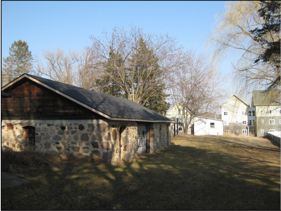
Old barn and house with 2009 FlynnTown Apartments next door.
