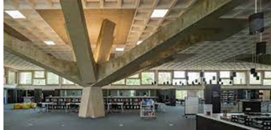
SJU Alcuin Library interior – renovated 2016
