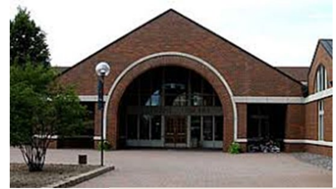
CSB Clemens Library entrance
