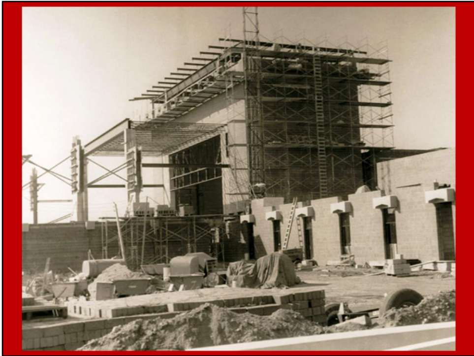
http://cdm.csbsju.edu/cdm/ref/collection/SBM/id/506 SBM.20a02 Benedicta Arts Center (BAC)" Construction
