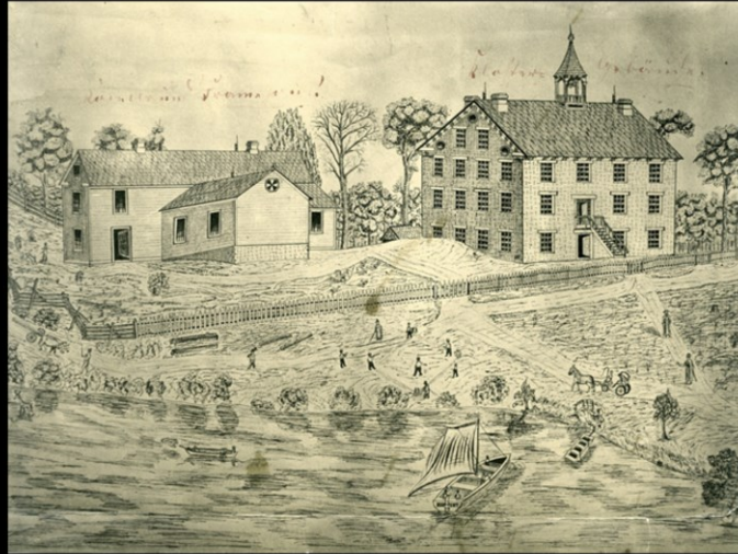
Drawing of the “Frame House” (left) and the “Old Stone House” (right)
